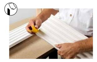
• Lightly sand the cut edges with sandpaper and remove the dust.
