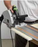
• Cut the panels to fit (Hand saw with set beam or circular saw with rail).
