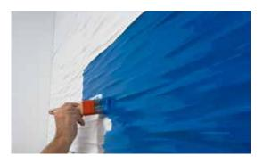
• If final painting has not been undertaken before assembly, apply the final coat of paint to the panels after drying (approx. 6 hours) and within 4 weeks (see FINISH).
