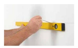
• Align and mark the lower laying line with the spirit level.
