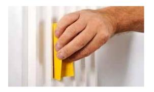
Allow the glue to dry (min. 6 hours) then sand the outsides of the joints lightly (sandpaper 150 grit or less) and retouch them again with ADEFIX<sup>®</sup> adhesive.
